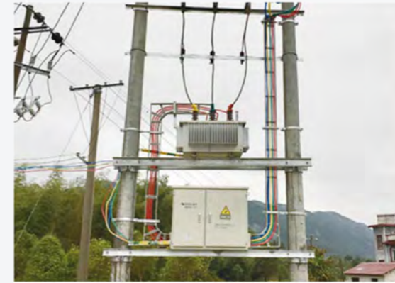
Power Distribution Network Project
