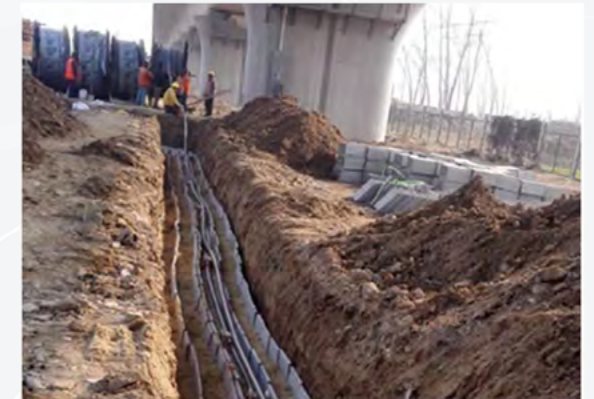
Power Cable Project
