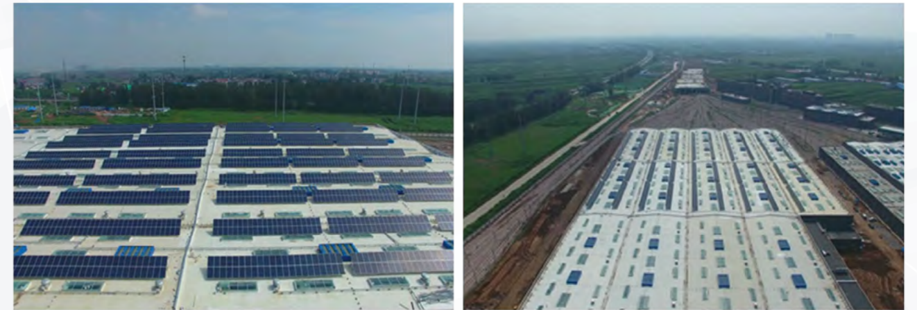
The first national MW subway photovoltaic project
